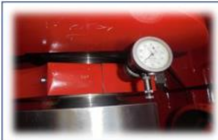
Web deflection inspection
