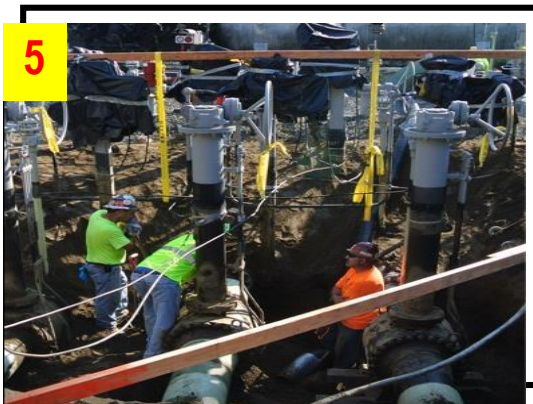
5 Exavation in refinery
