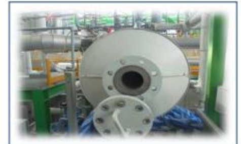
S/D damper inspection
